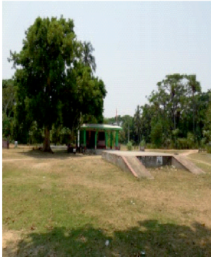
Fig. 9.a: Nagasapur present shed
